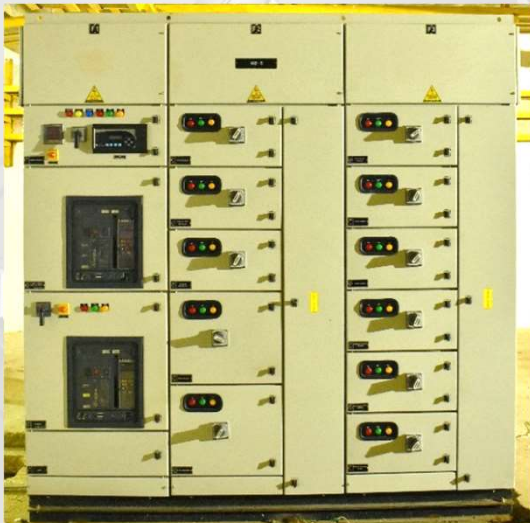
UNIT AUXILIARY BOARD PANELS
