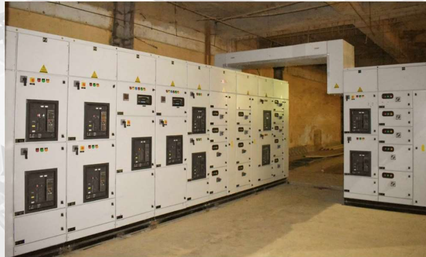
STATION SERVICE BOARD PANELS
