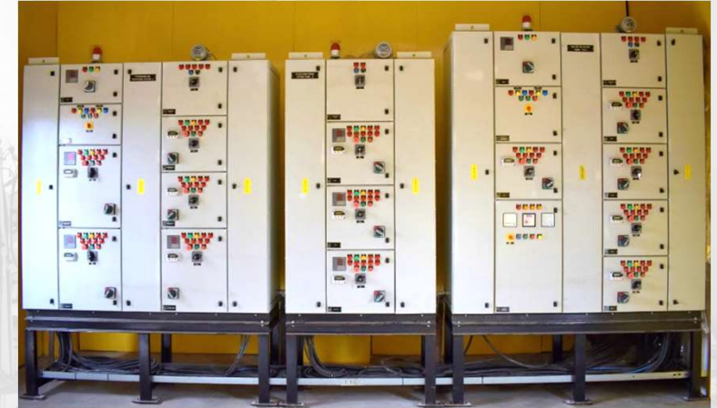
CONTROL PANEL FOR 19 SUBMERSIBLE PUMPS
