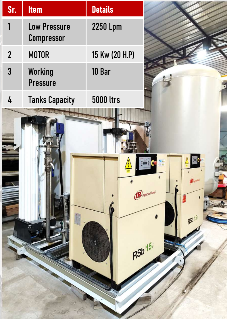
DUAL SCREW COMPRESSOR AIR SYSTEM WITH AIR DRYERS, AFTER COOLER & TANK (5000 Ltrs)
