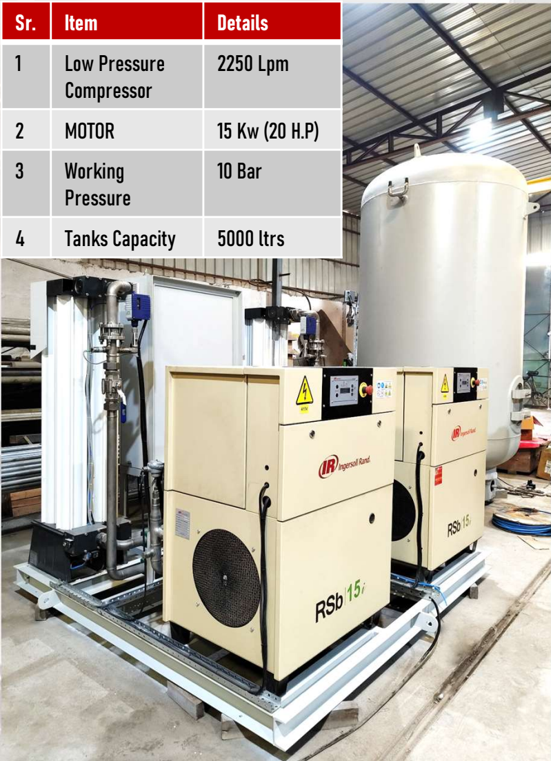
DUAL SCREW COMPRESSOR AIR SYSTEM WITH AIR DRYERS, AFTER COOLER & TANK (5000 Ltrs)
